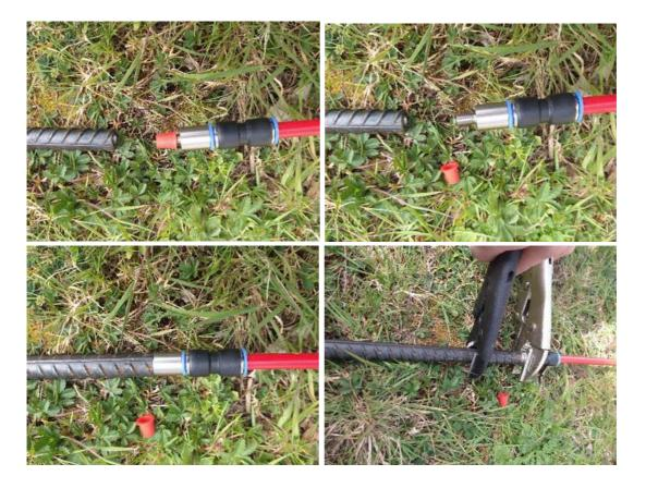
Uncoil the vent tube and attach it to the deepest anchor so that it protrudes 300mm beyond the end of the anchor.
