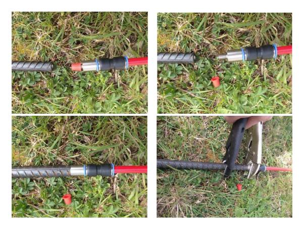
Uncoil the grout tube and attach it to the end of the deepest anchor.
