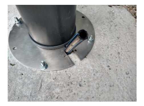
If using the resin fixing kit insert the fixing into the holes in the securing plates and secure in place using the nuts and washers.
