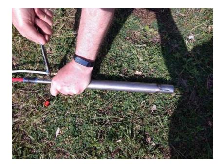
Using adhesive tape secure the hydraulic tubing to the anchor protective tube at regular intervals.
