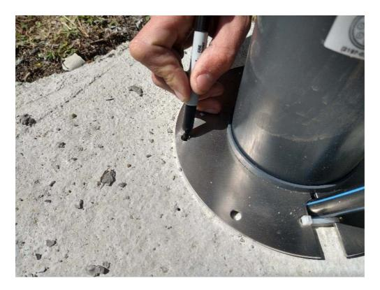
Drill the holes as required by the fixing type.
