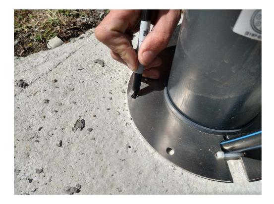
Drill the holes as required by the fixing type.
